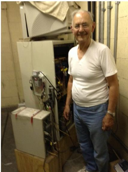
Seen in the left picture is one of the Technical Committee members, Phil, W8PSK, installing a new 12V power system with smart battery backup for repeater receiver, controller and APRS units in the Offenhauer Penthouse. A detail of the set up is shown on the right.
