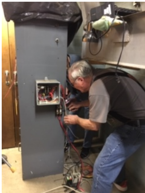
Bob-WB8NQW rewiring link between rcvrs and xmtrs. No more telephone lines!
