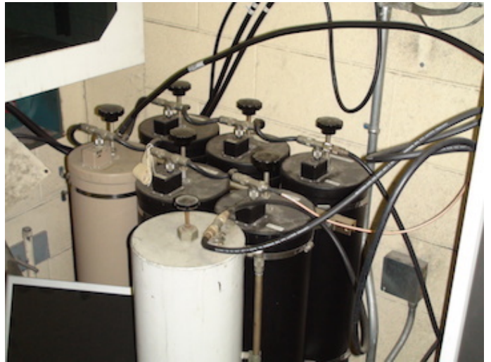
VHF duplexers (cans). UHF duplexers are in the rcvr rack
