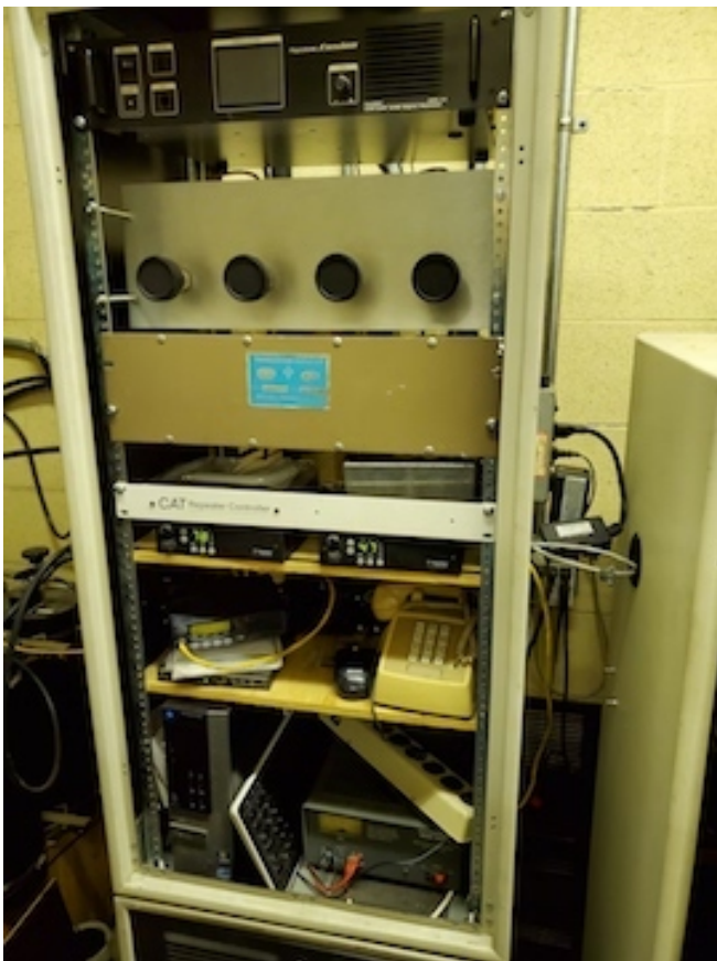
Existing rcvr rack. VHF and UHF rcvrs on shelf above telephone; then CAT controller, UHF duplexers and fusion repeater.
