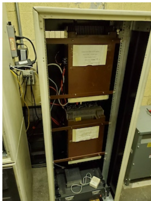
New xmtr rack with GE Master VHF and UHF units installed—power supply on bottom
