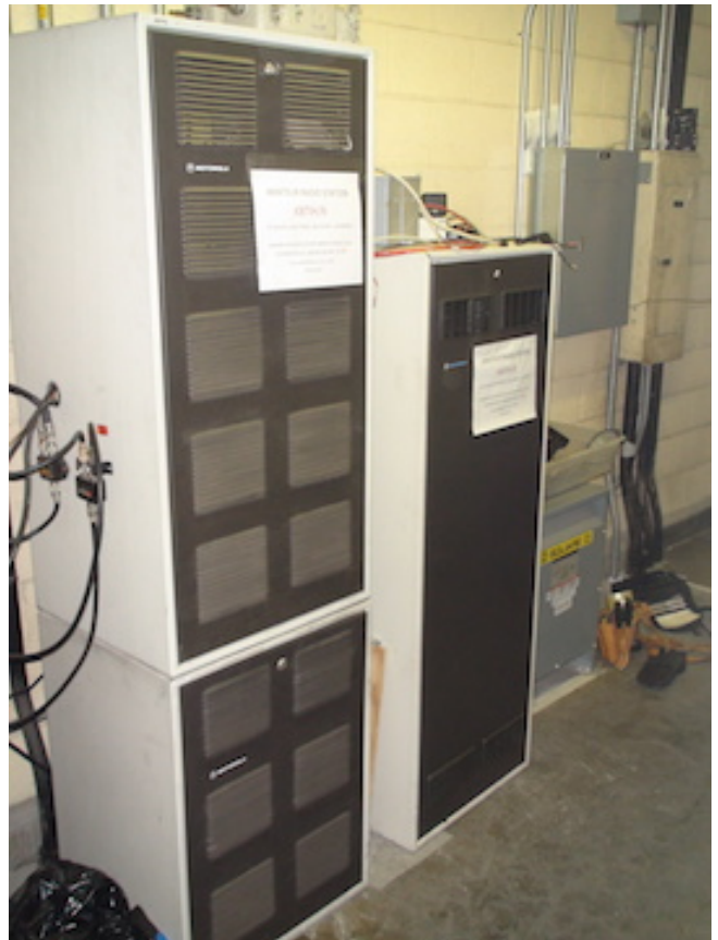
Final assembly—rcvrs on left and xmtrs on right. Duplexers on left of rcvr rack used to combine VHF and UHF signals to feed dual band vertical antennas on the roof
